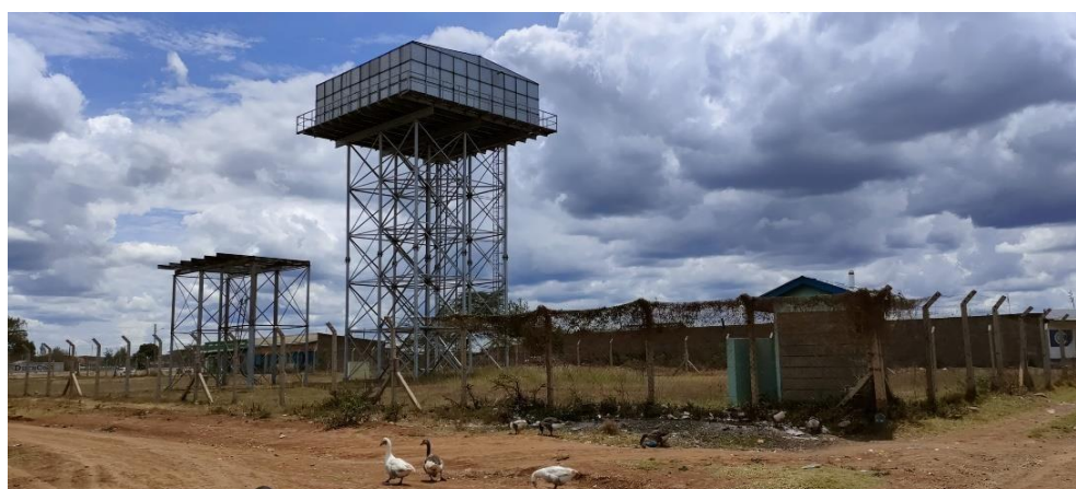
An elevated water tank at NYAHUWASCO site
