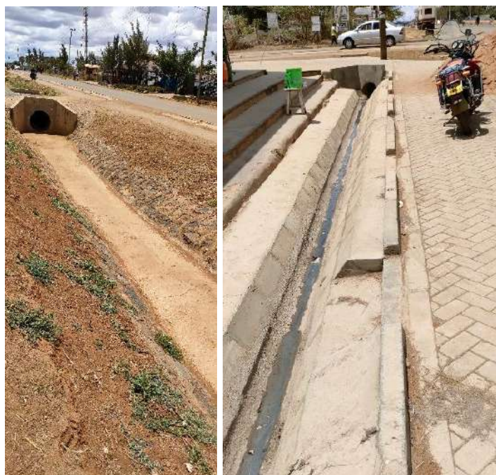
Plate 2-21: Open storm water civil drains within the CBD
