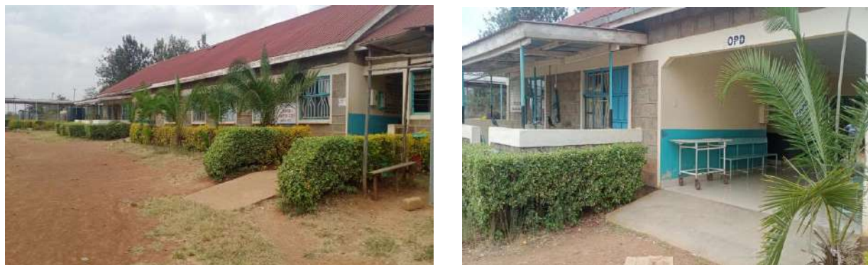
Plate 2-24: Rumuruti sub-county hospital out-patient department
