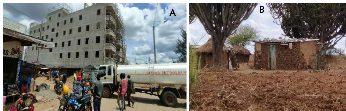
Plate 2-15: Typical housing units in African location (A) and Muthaiga estate (B)
