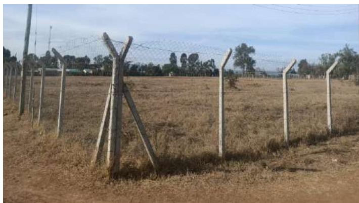
Plate 2-28: Existing Rumuruti stadium
