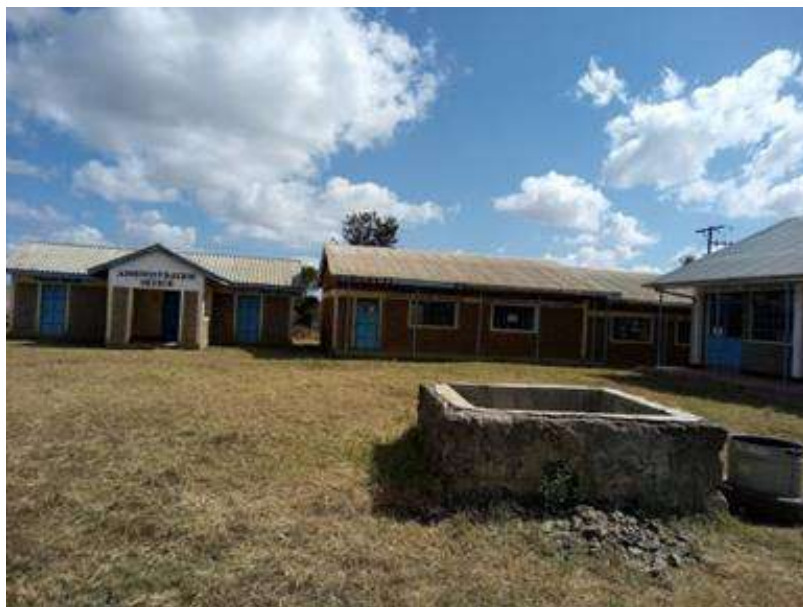
Plate 2-27: Rumuruti Vocational Centre
