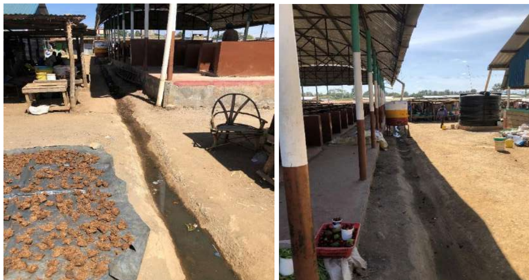
Plate 2-8: Shallow open drains in the market
