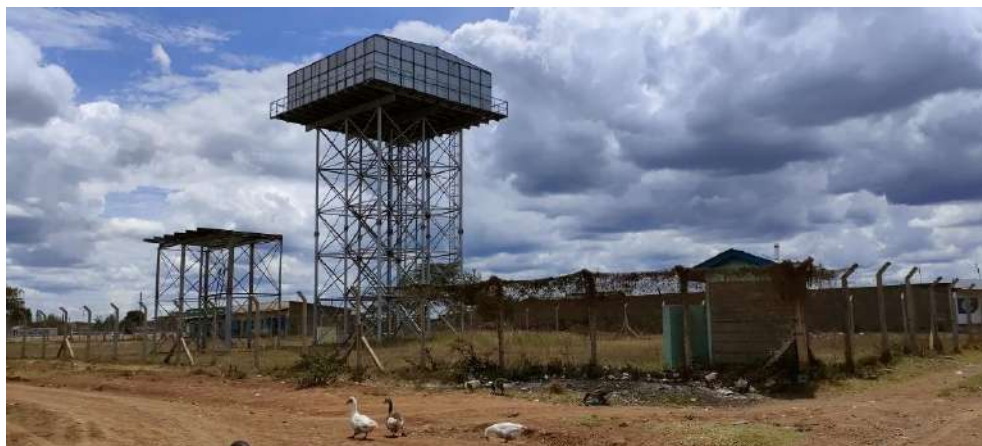
Plate 2-22: An elevated water tank at NYAHUWASCO site
